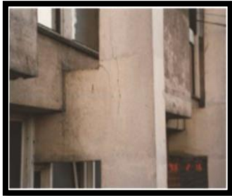
Figure 5.1.6: CORROSION IN R.C.C.
